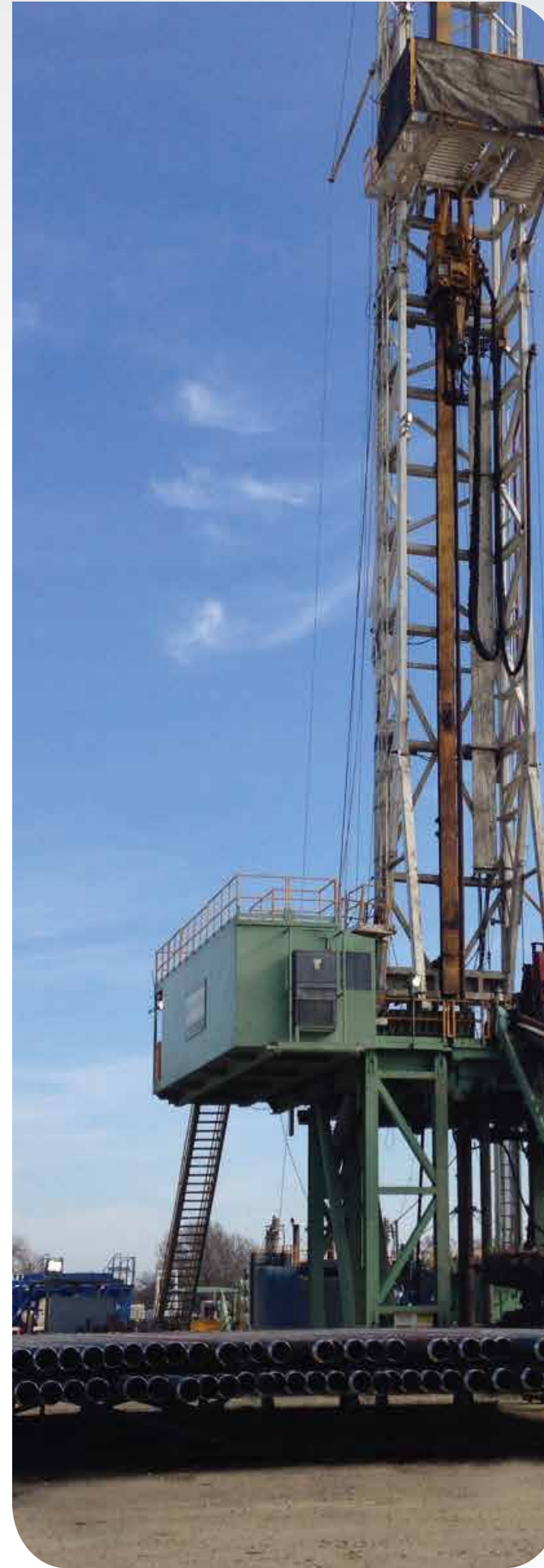
Our products on site
